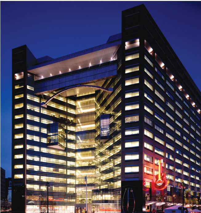
Compuware's headquarters has a system that combines a variable volume, low-temperature primary air supply system with underfloor air-distribution.
