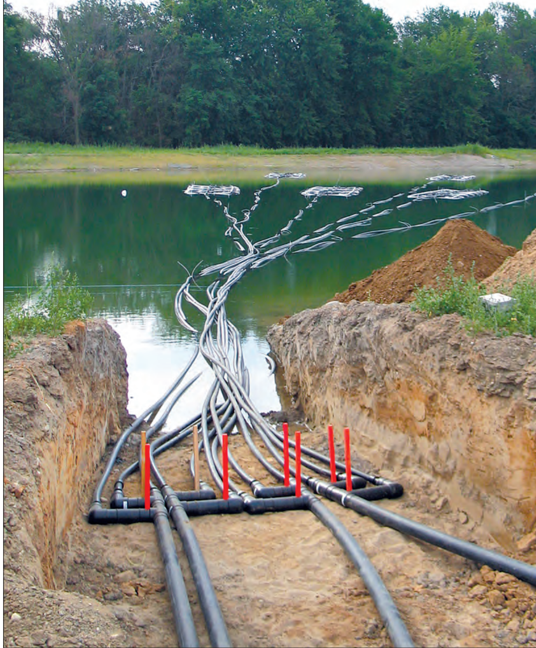
One third of the geothermal system's piping coils are in the pond. Attaching weights and filling the coils with fluid keeps this aquatic geothermal system submerged and in place.
